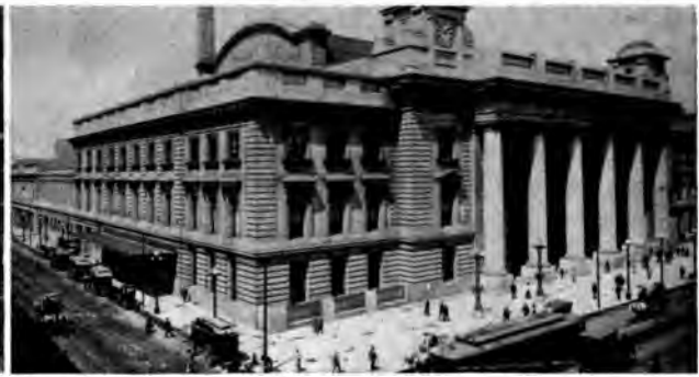
Chicago & North-Western Terminal, Chicago, 600,000 square feet Sarco No. 6 Waterproofing, 225,000 square feet Sarco Flooring.
